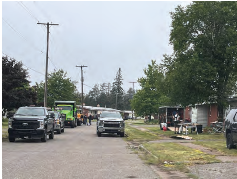
Sawyer Village under construction.
