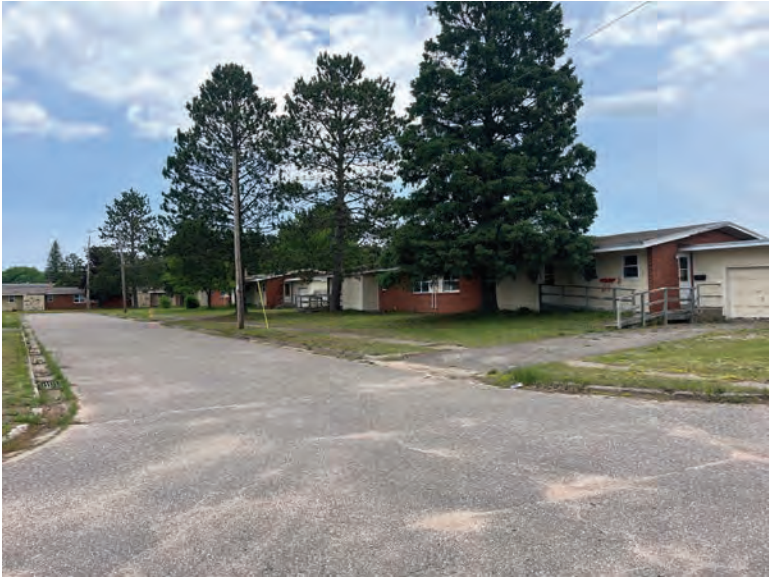
Sawyer Village homes before renovations.
