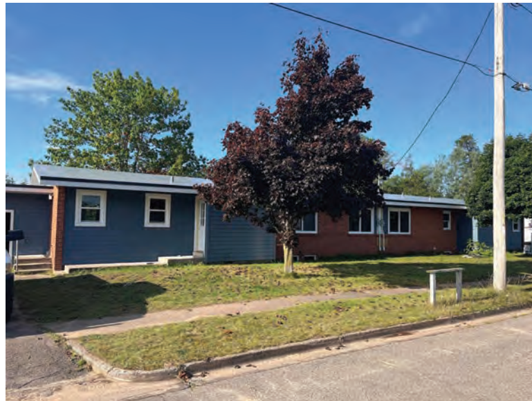
Sawyer Village homes after renovations.
