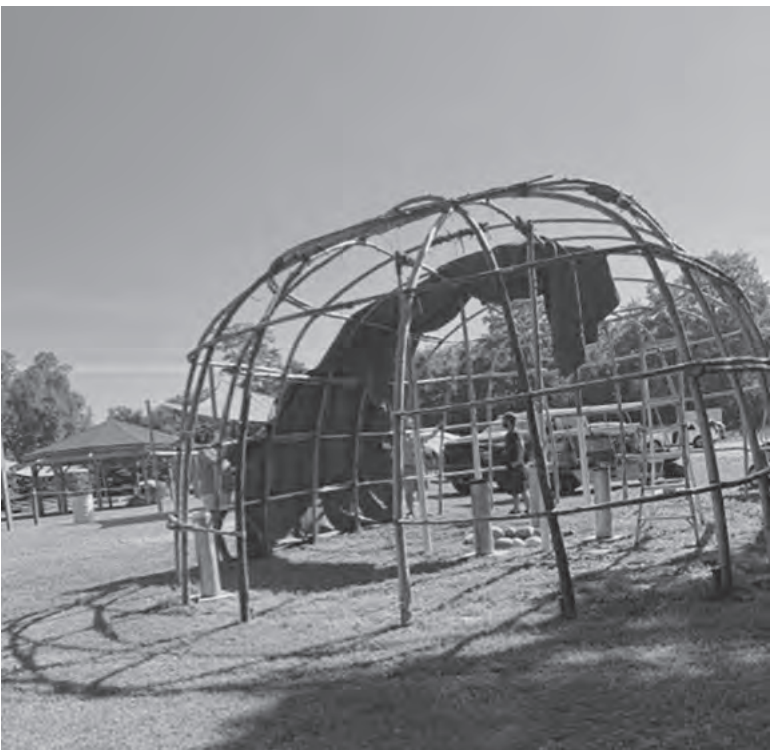
The community came together to build a new teaching lodge in Hessel.
