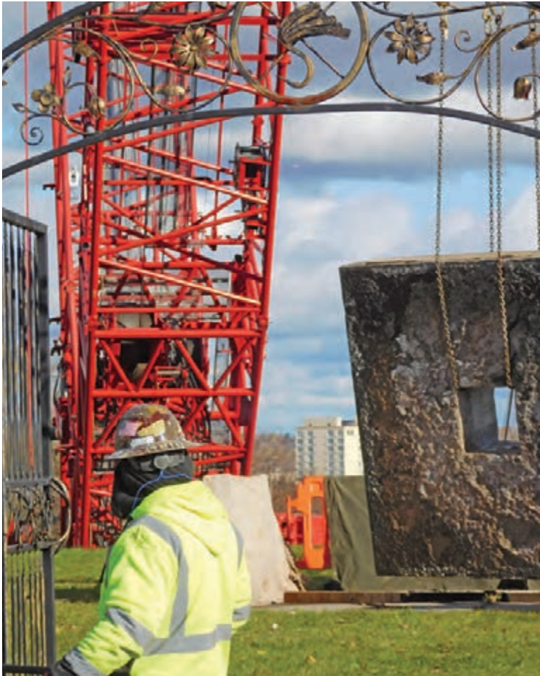
The base of the obelisk being removed.
