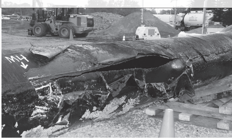
Enbridge Oil Pipe Line Burst at the Kalamazoo River from 2010. When
